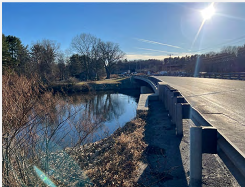
Photo 6- Washington Street Crossing of the Little Androscoggin River
