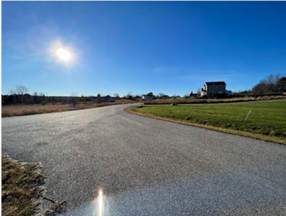
Photo 2 - Lubear Way Potential Pump Station Location
